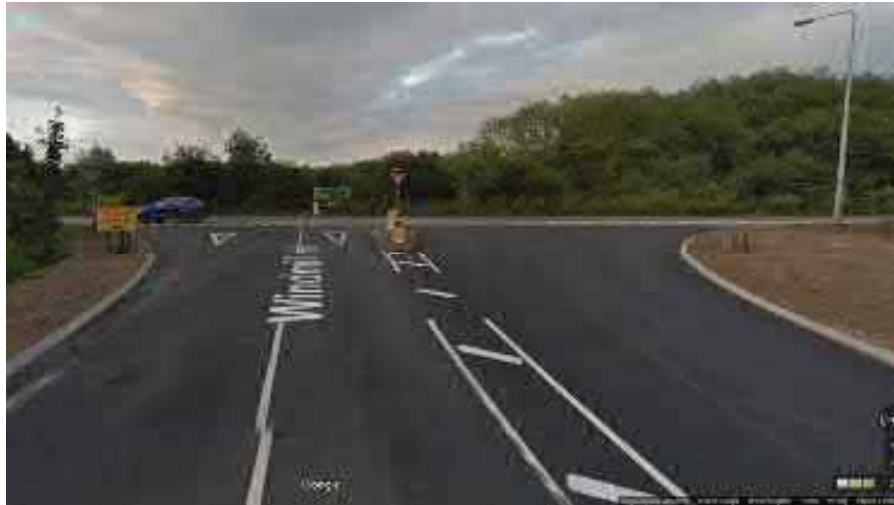
Figure 7: Google Street View Windmill Hill Road/A142 Fordham Road T-Junction
