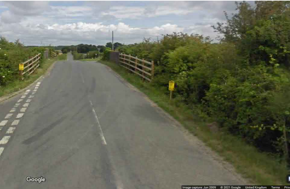
Figure 32: Google Street View of the Bridge
