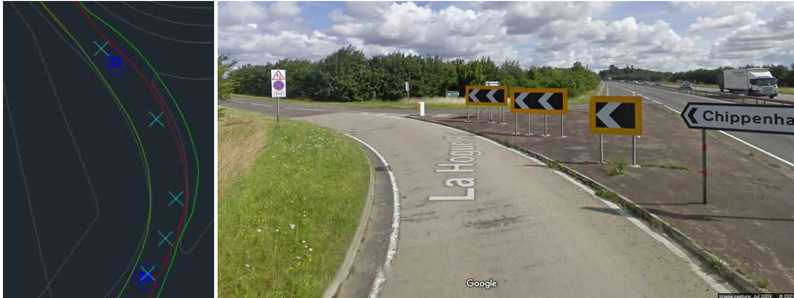
Figure 51: Swept Path Analysis: 1000T Crane Figure 52: Google Street View A11 Northbound Off-Slip onto La Hogue Road
