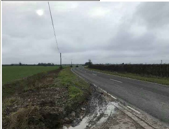
Site Visit Photo: View Left
