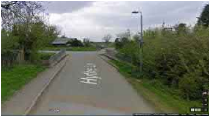
Figure 29: 1000T Crane Entry Hythe Bridge
