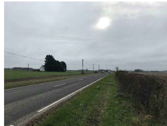
Site Visit Photo Existing Site Access View: Right
