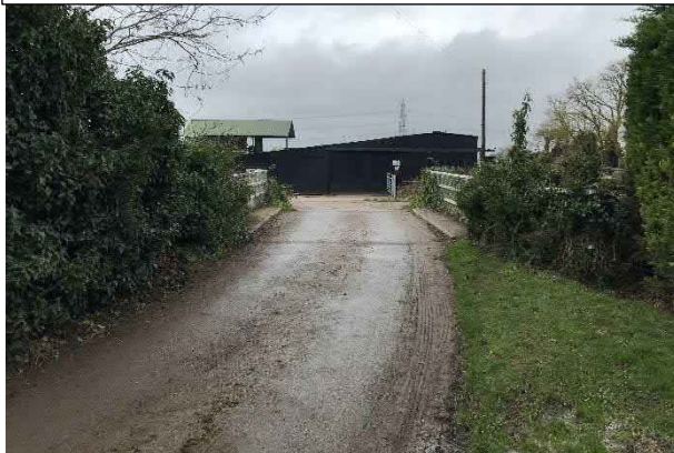
View of the bridge to the farm from Anchor Lane
