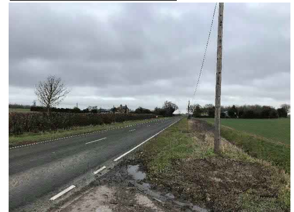
Site Visit Photo: View Right
