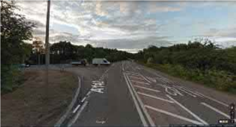
Figure 3: Google Street View of A142 Fordham Road/Windmill Hill Road T-Junction
