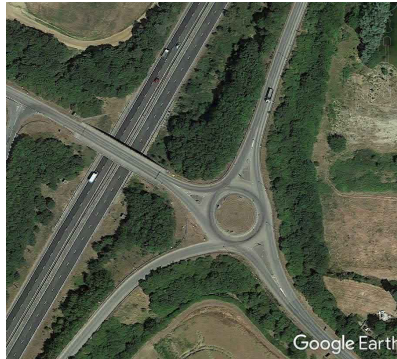
Figure 44: Dane Hill Roundabout Google Earth Aerial Photo*
